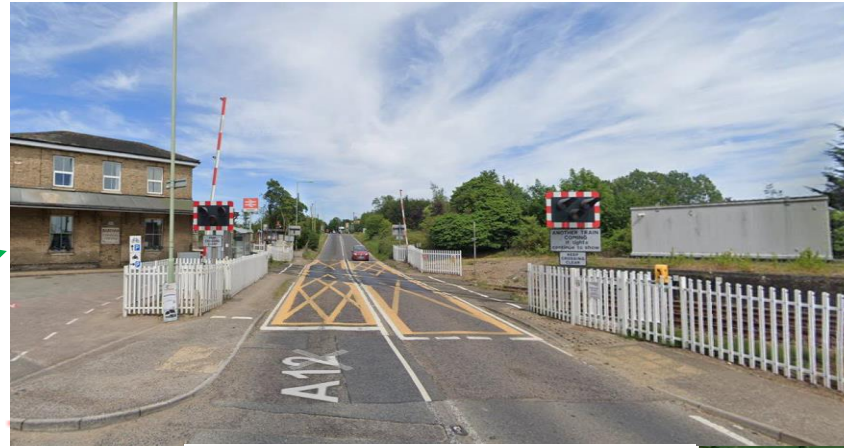
Darsham Level Crossing
